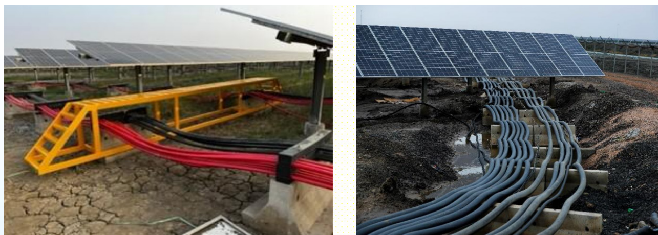
Figure 3: DC and AC cables installed above the ground with colour coding
