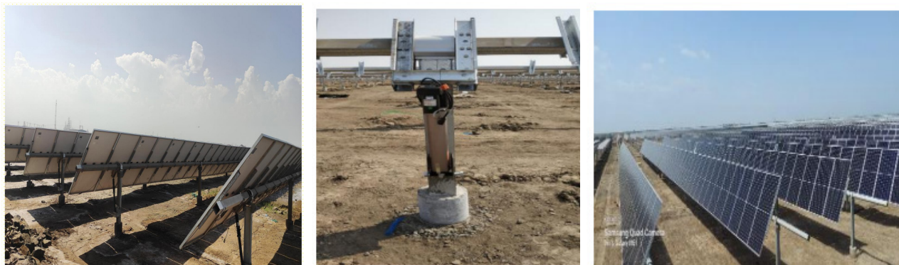
Figure 4: Tracker based ground mounted solar power plants
