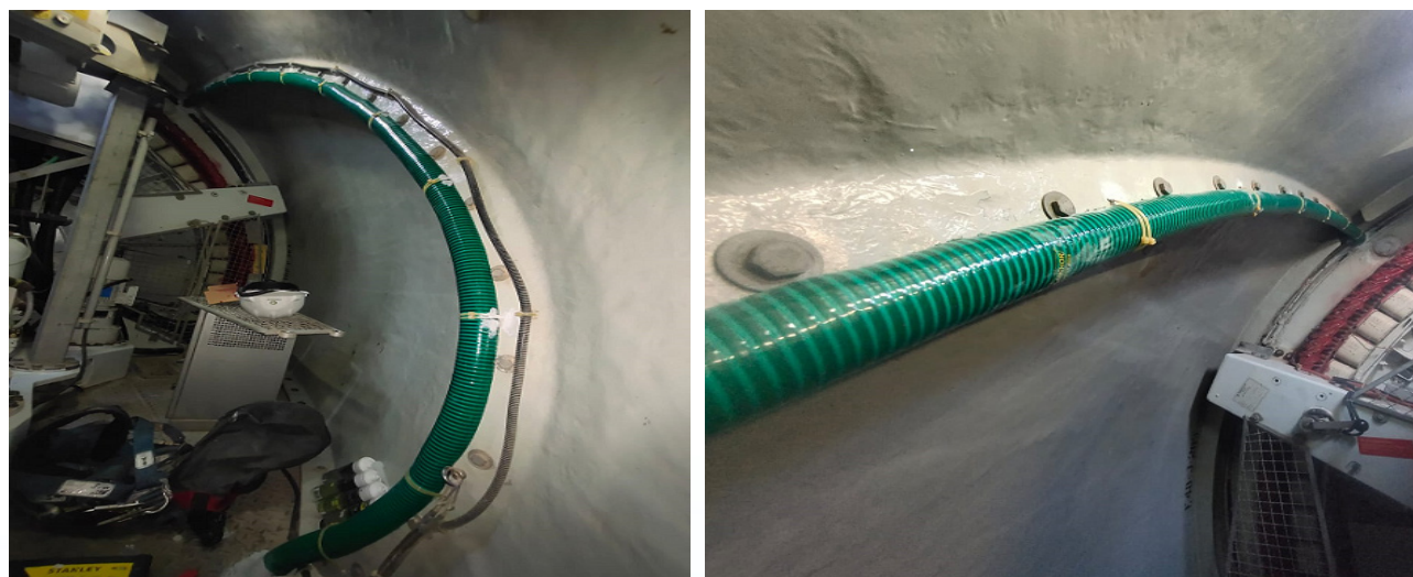
Figure 16: Water drainage hose pipe fitment at nacelle Glass Reinforced Plastic (GRP) joint
